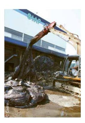
Destruction of oil, oily sand, oily debris, oiled fauna by thermal treatments at high temperatures in industrial plants (incinerators, cement plants), by incineration (combustion with oxygen) or by pyrolysis (with low oxygen). For both of these, the volume of waste is reduced by up to 90 % and residues must be disposed of in industrial landfill.
